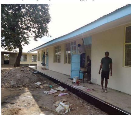
we wanted to start looking towards one of the last important problems – the rain water. At first we wanted to level the ground in even hight compared to the tiles. We also wanted to mix the soil with cement to prevent the foundation to get washed-out. But that won't be enogh to protect the building from water and mud, because the whole ground is leveled down towards our building. We thought it might make most sense to build a small concrete channel leading mud and water around the building
