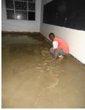
used a substandard cement, which was not hard and stable enough to apply tiles on it.
